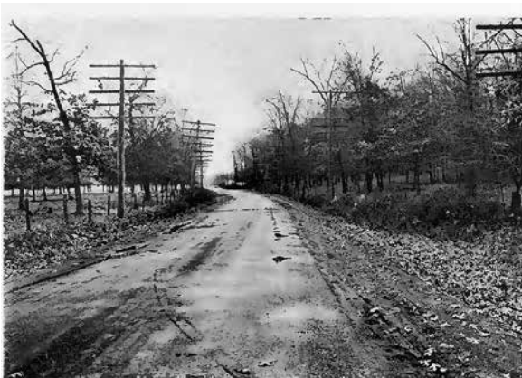
THE “IDEAL SECTION.” SITE BEFORE IMPROVEMENT
