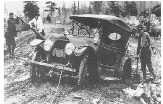
Figure 2. Image illustrating poor condition of many early-twentieth-century roads. 12
