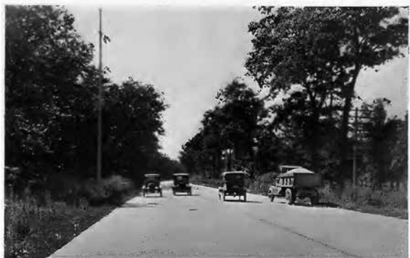
A COMPLETED PORTION OF THE “IDEAL SECTION”
