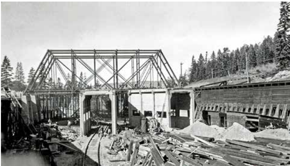
Construction of the Norden snowsheds circa 1923
