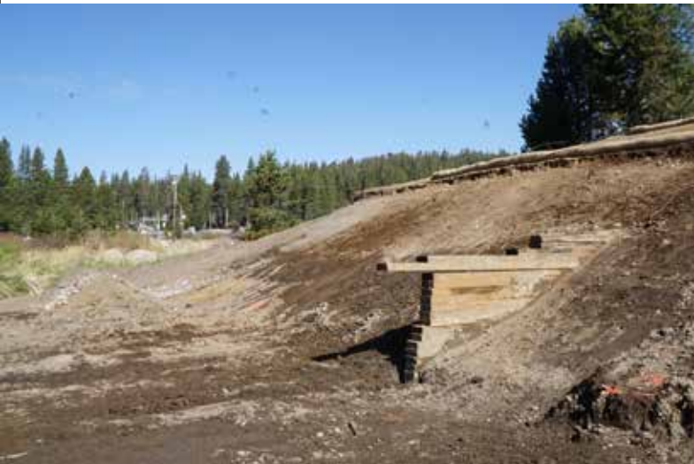
Above and below, more old dam remnants exposed after the second notching of the old dam to let out all remaining water. The old redwood showed no signs of rot.
