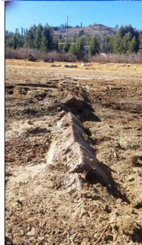
more views of what may be the old dam poking out of the mud after the second notching released remaining water from what had been Lake Van Norden.
