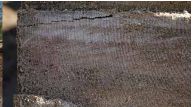
Above and below, more old dam remnants exposed after the second notching of the old dam to let out all remaining water. The old redwood showed no signs of rot.
