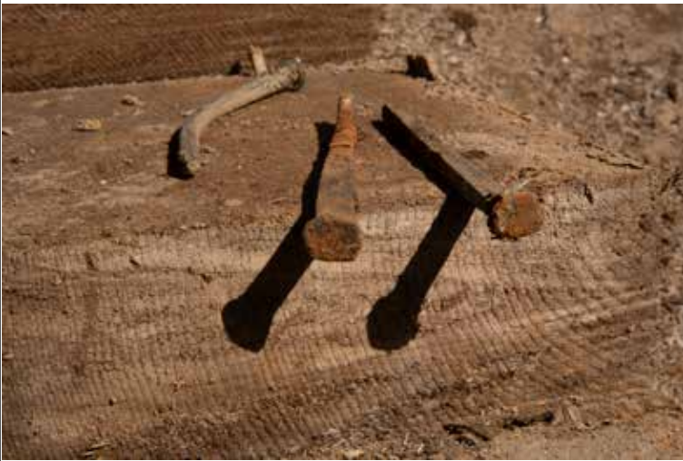
Above and below, more old dam remnants exposed after the second notching of the old dam to let out all remaining water. The old redwood showed no signs of rot.
