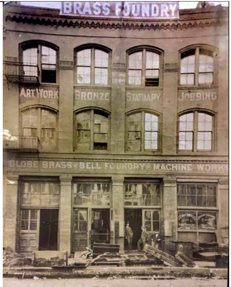
This Globe foundry in San Francisco predated the Oakland foundry. It appears that this photograph may show some of the earthquake damage that prompted the move across the bay.
