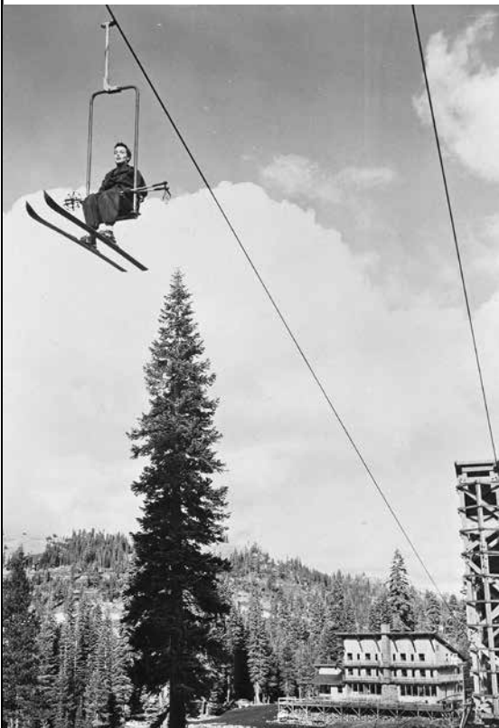
Sugar Bowl Lodge in the background. First chairlift in California was a single seater.
