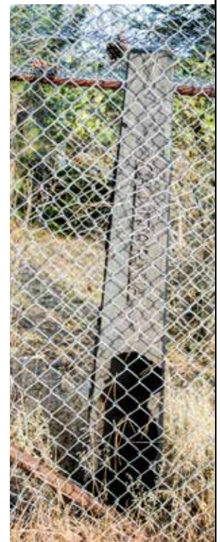
Marker for the Von Schmidt Line, his surveyed border between California and Nevada outside of Verdi, Nevada. Top left says, "120° west of Greenwich."
