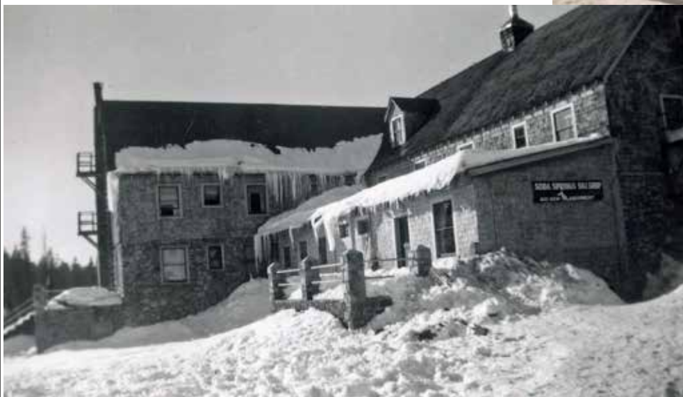
Above, the rear of the Soda Springs Hotel, 1947. The sign on the end of the building says, "Soda Springs Ski Shop."
