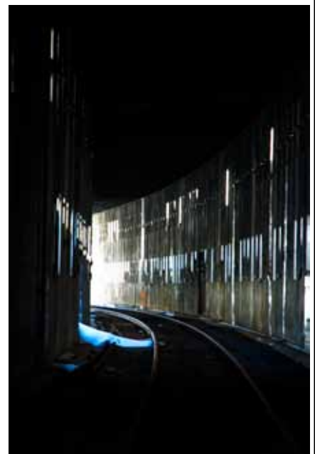
Left: Picture of a signal in the sheds just above the entrance to the tunnel that went down to the commissary.
