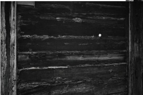
To the left you can see a close up of the siding which is composed of Southern Pacific snowshed timbers made available when the snowsheds were rebuilt in the late 1940's.
